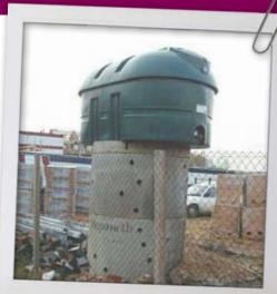
How not to install an oil storage tank!
