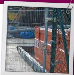
Secured fuel tank in secondary containment
